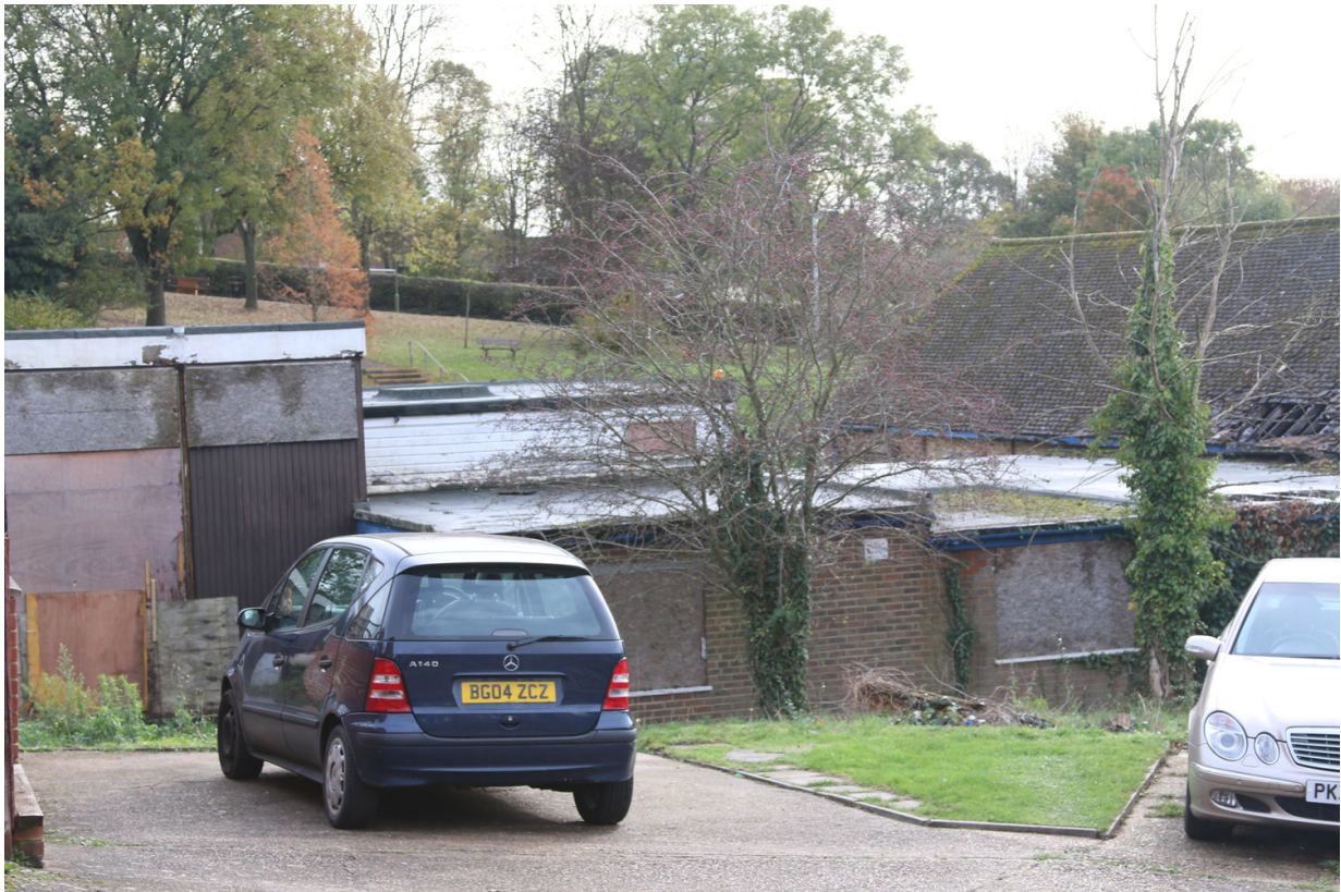
Rear of building – view from Fairway Court
