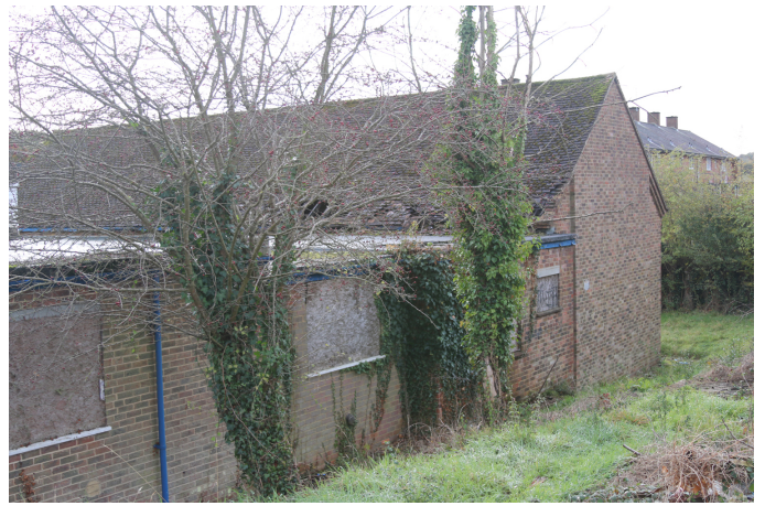
Land falls away at rear of building
