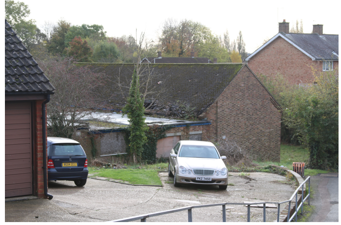
View from Fairway alley at rear
