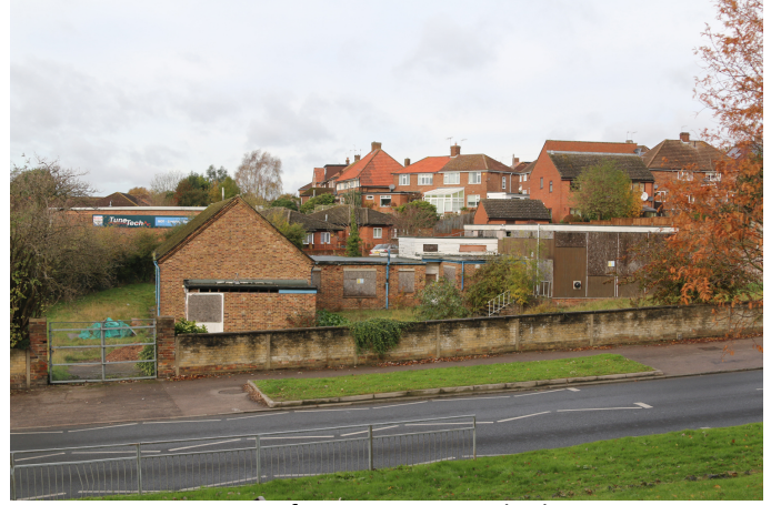
View from Georgewood Rd
